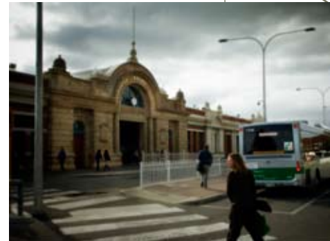
Stage one of the Fremantle Station facade restoration was completed.
