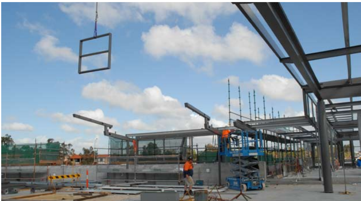
Station construction at Bull Creek was well under way.
