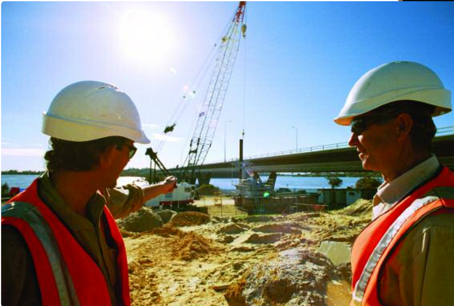
Work under way at Mt Henry Bridge.
